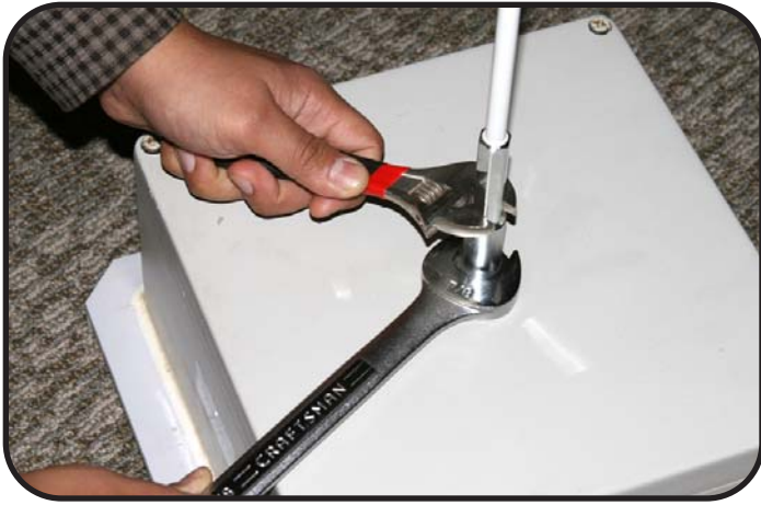
Remove Monopole Whip (Use a second wrench with opposing force to prevent monopole fitting from unscrewing)
