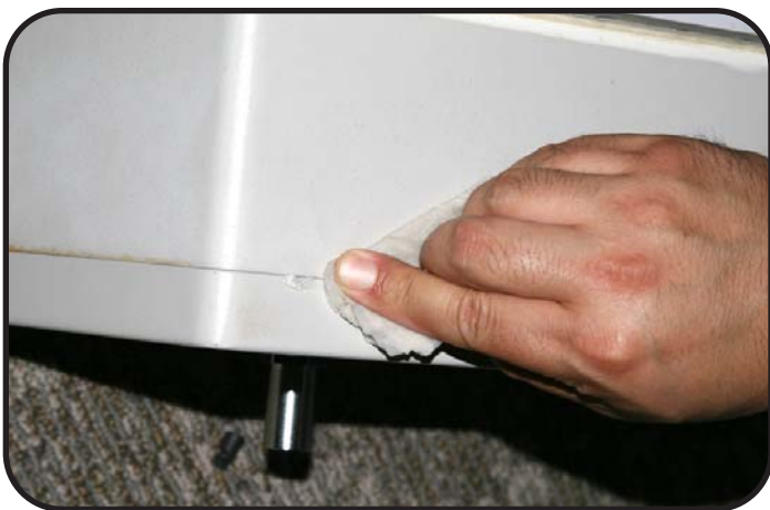
Wipe off the excess caulk
